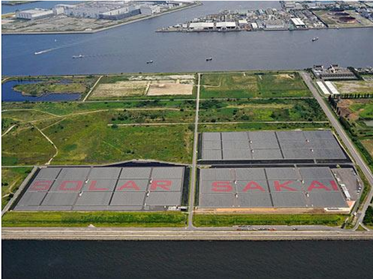
Large-scale solar power plant (10MW by KEPCO since 2011)
