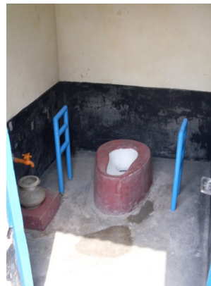
Toilet built for people with a disability in Dhaka, Bangladesh. Credit: Juliet Willetts
