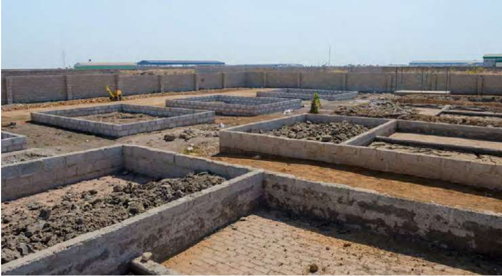
Kanyama FSTP decommissioned sludge drying beds
