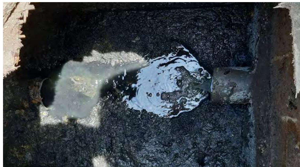
Inlet of the DEWATS
