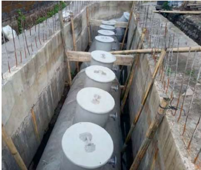
Installation of DEWATS technology
