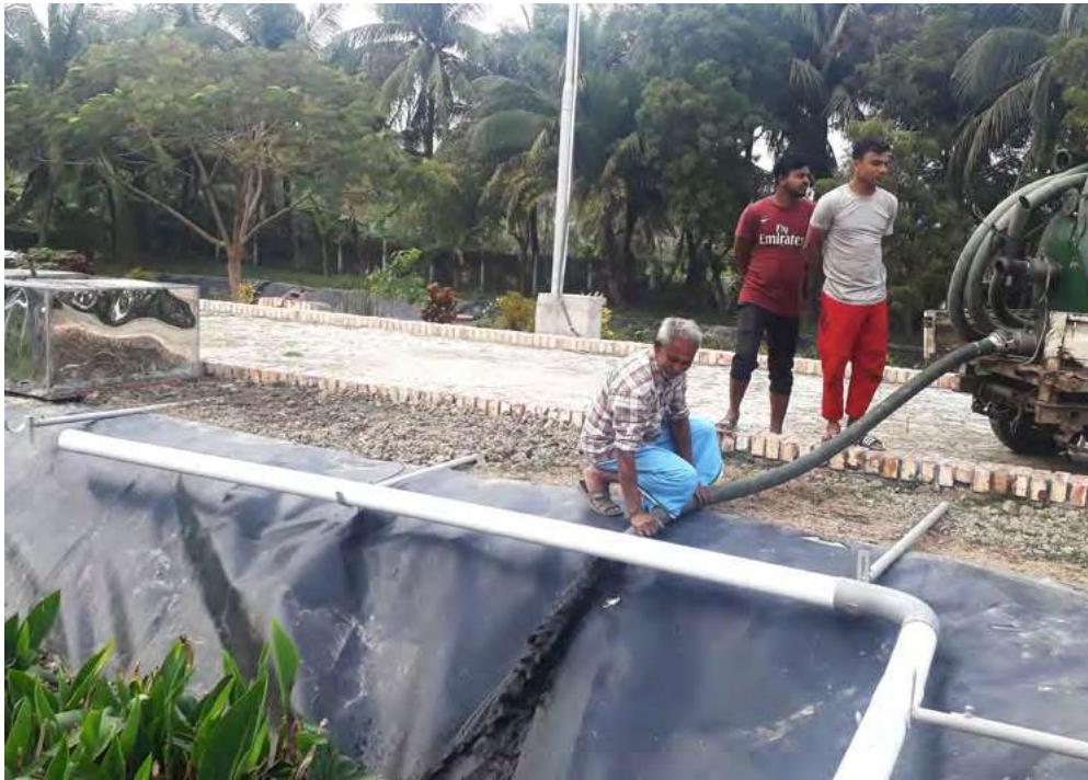
Operators discharging influent directly to planted constructed wetland bed
