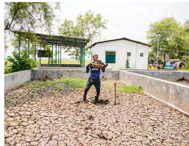
Removing dried sludge from the drying beds
