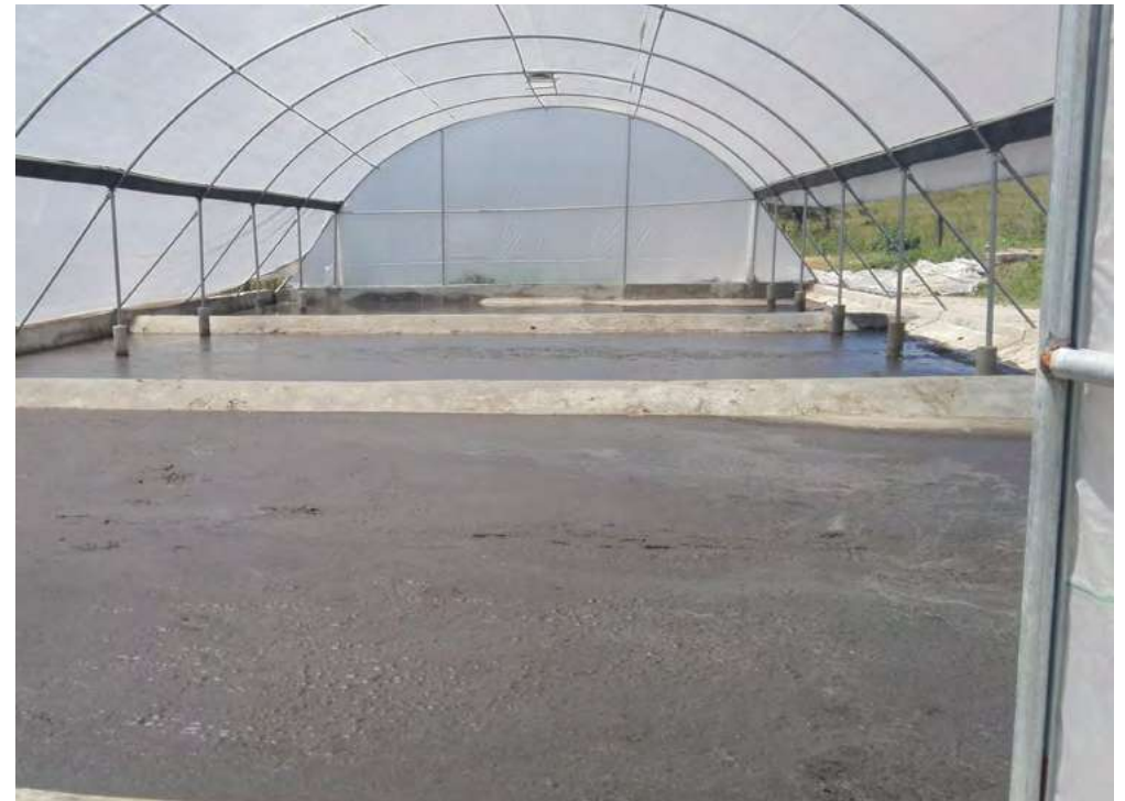
Solar dryer in the NAWASSCOAL facility
