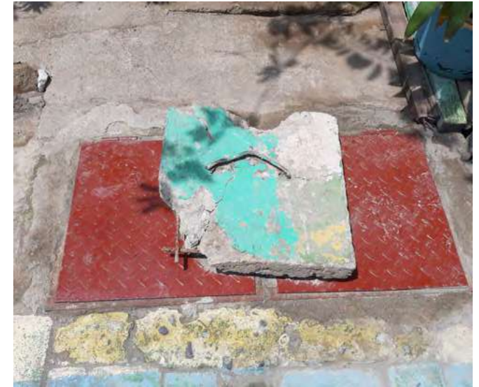
Comparison of concrete and lightweight iron cover for inspection chamber cover
