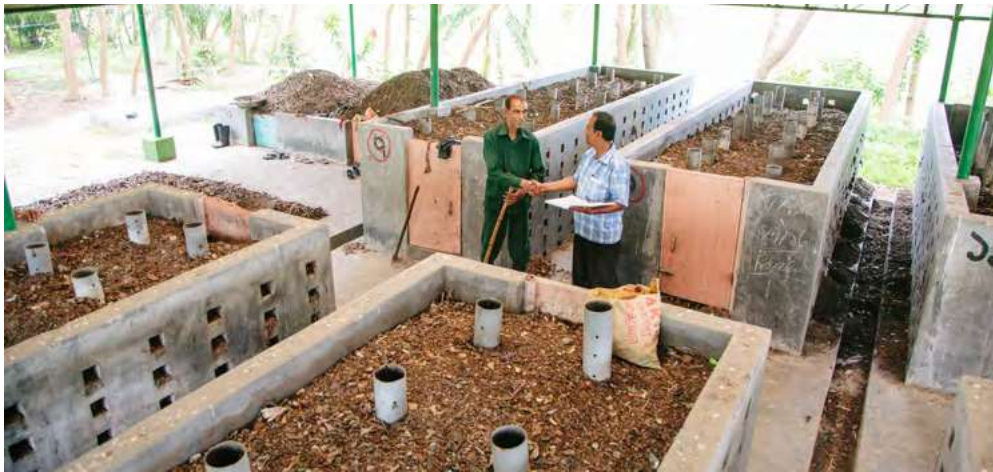
Co-composting of treated sludge and organic waste
