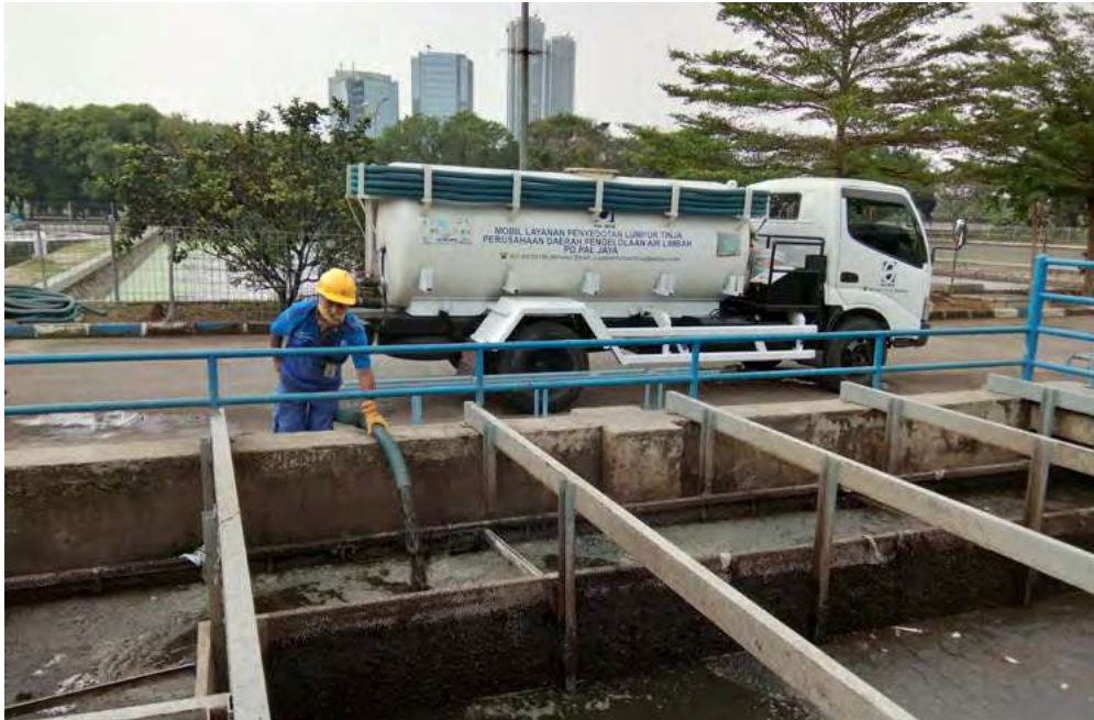
Conventional aerobic pond
