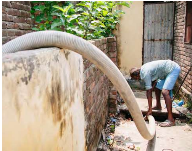
Desludging household containment
