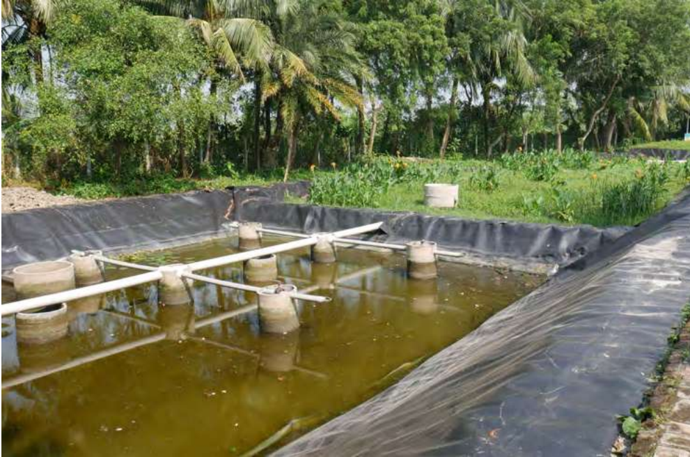
BOD levels of treated water are significantly lower than canal water beside the FSTP
