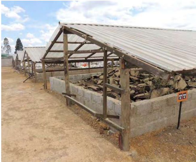
Roofed sludge drying beds at Kanyama FSTP
