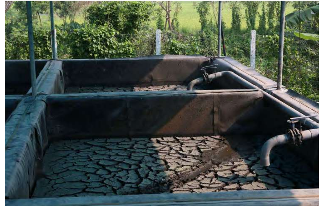
Sludge drying beds
