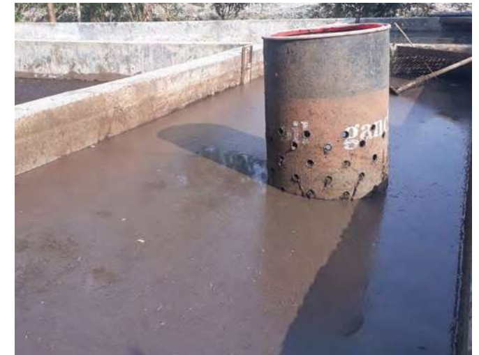
Settled sludge moves to the natural drying bed via the filtering gate
