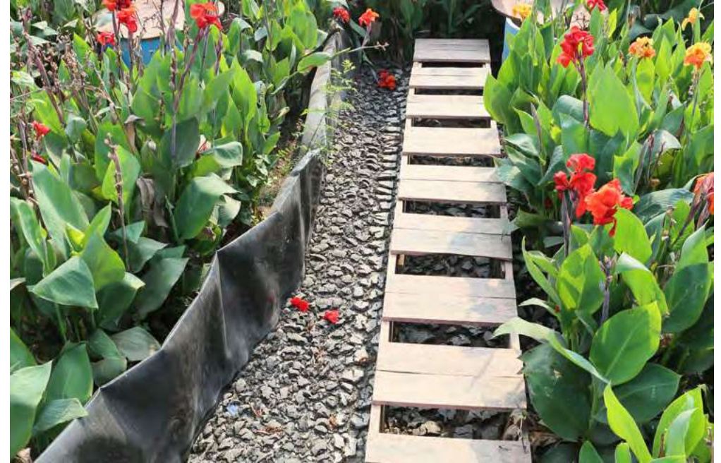
Dried sludge in planted constructed wetland
