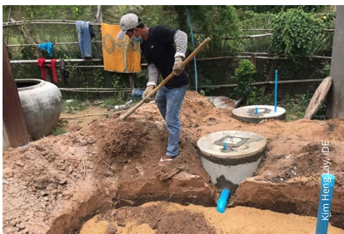
The All-Season Upgrade product, a climate-resilient technology for areas that experience seasonal flooding, high groundwater and low soil infiltration, designed and tested by iDE in collaboration with Engineers Without Borders Australia.
