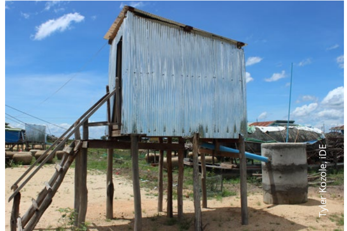
Trapeang Chan commune, Kampong Chhnang province, Cambodia. Elevated latrines are an aspirational product for families living in flood-prone areas. iDE and Causal Design are teaming up to learn how to best provide targeted subsidies for similar, flood-resilient technology, with the intent of supporting vulnerable households in such environments to access sanitation.
