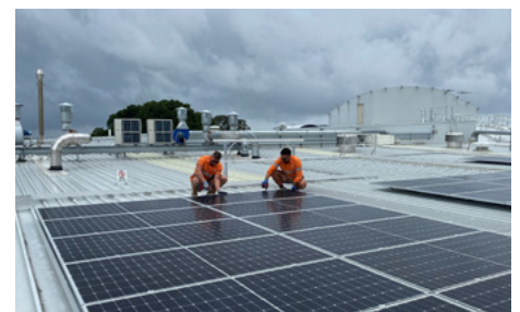
Solar cells being installed on the Botany Tech labs
