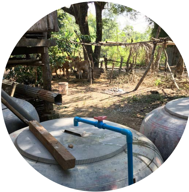
Rural water systems in Cambodia. Photo credit: Melita Grant
