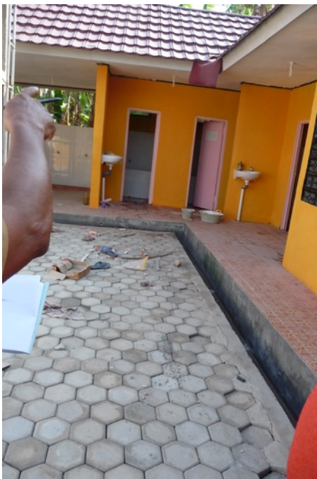
Figure 4-2: Newly constructed MCK++ has uneven paving and obstructed toilet doors.
