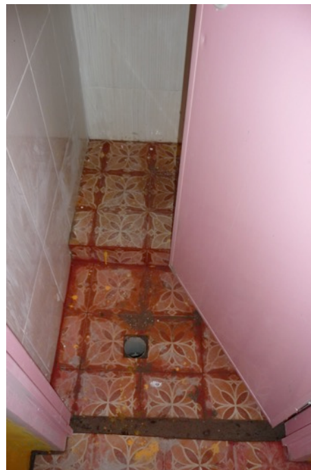
Figure 4-2: Newly constructed MCK++ has uneven paving and obstructed toilet doors.
