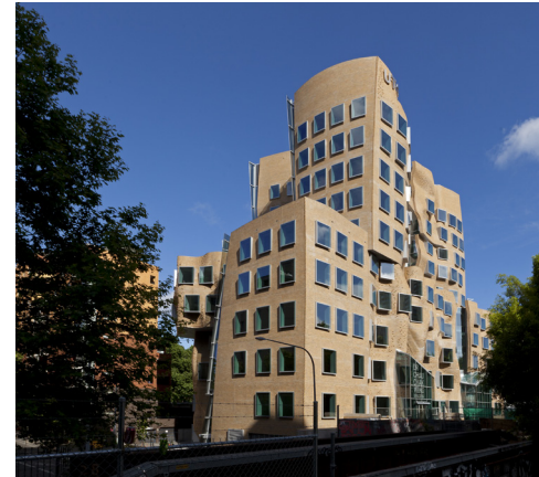
Exterior, eastern façade. Credit: Andrew Worssam
