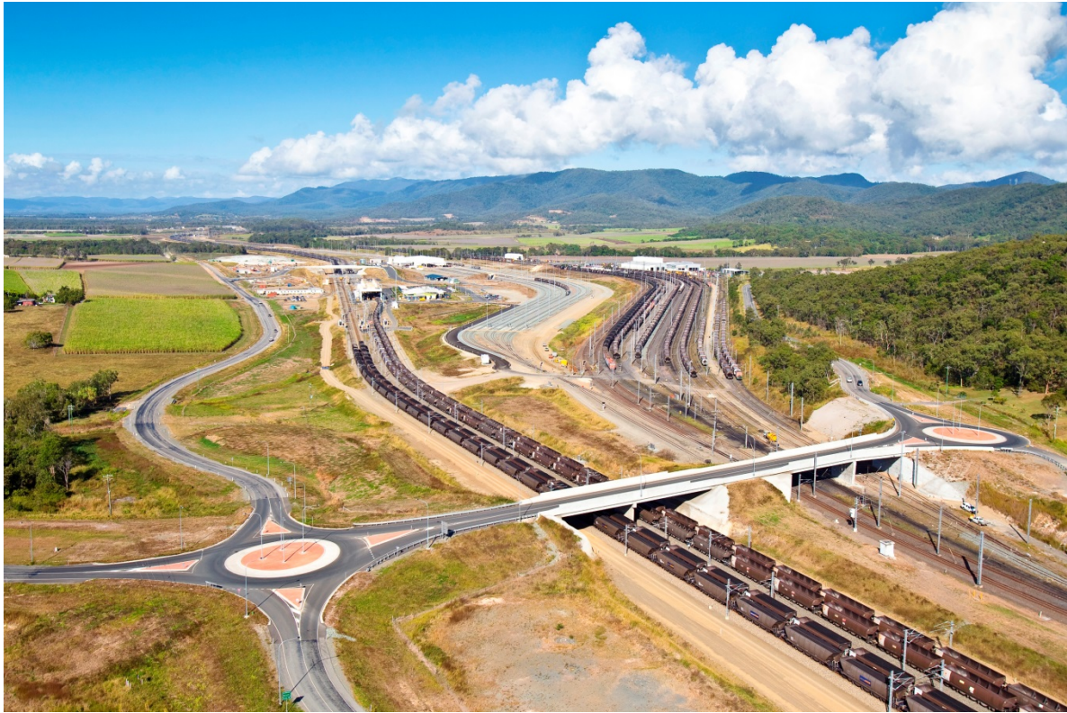
Figure 8: Jilalan Rail Yards near Sarina. Photo supplied by Mackay Regional Council.
