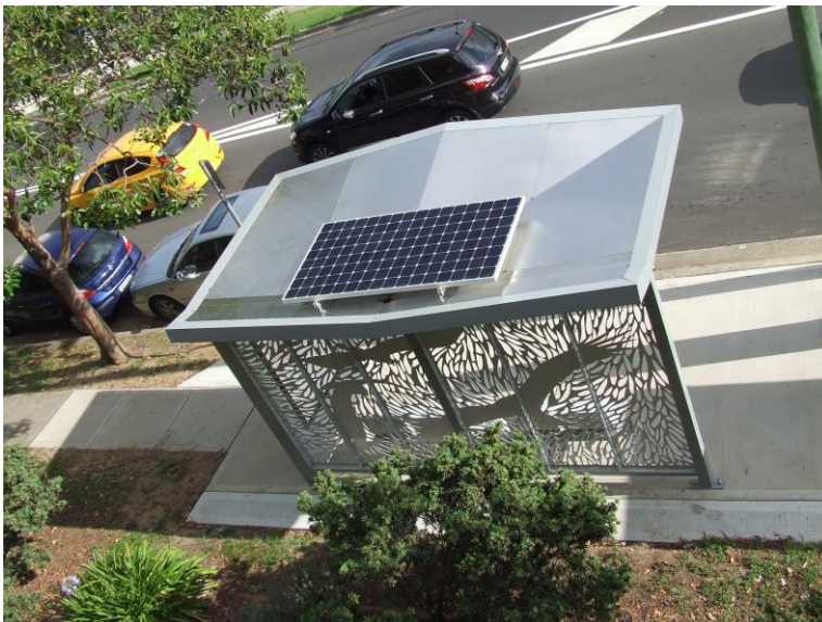
Figure 12. Solar panel installed on the roof of the CAPS prototype.
