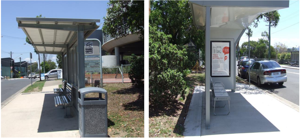
Figure 8: Side view of the two shelters (BS, left; CAPS, right) illustrating the differences in seat and roof construction and areas of shade.
